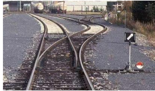
Fig 3.47 Railway switch
