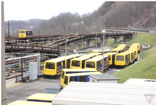
Fig 5.51 Depot in Morgantown Transit
