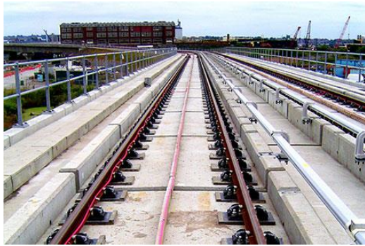
Fig 5.39 Steel rail on concrete base
