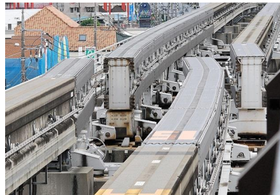
Fig 5.41 Switch of monorail
